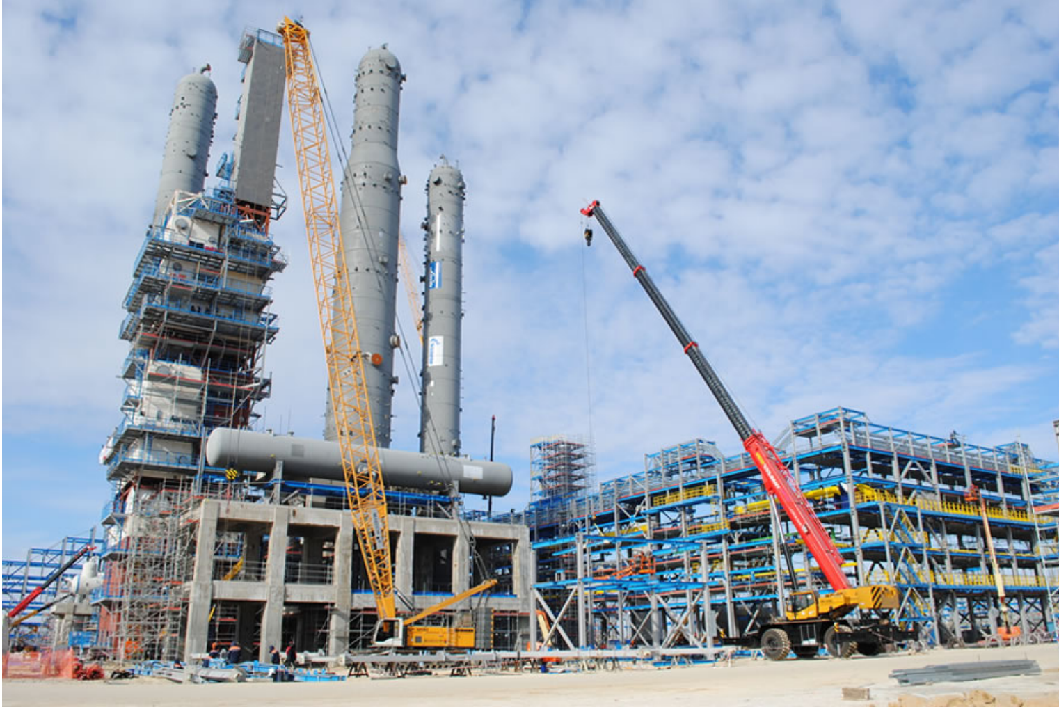
Amur GCC construction.
