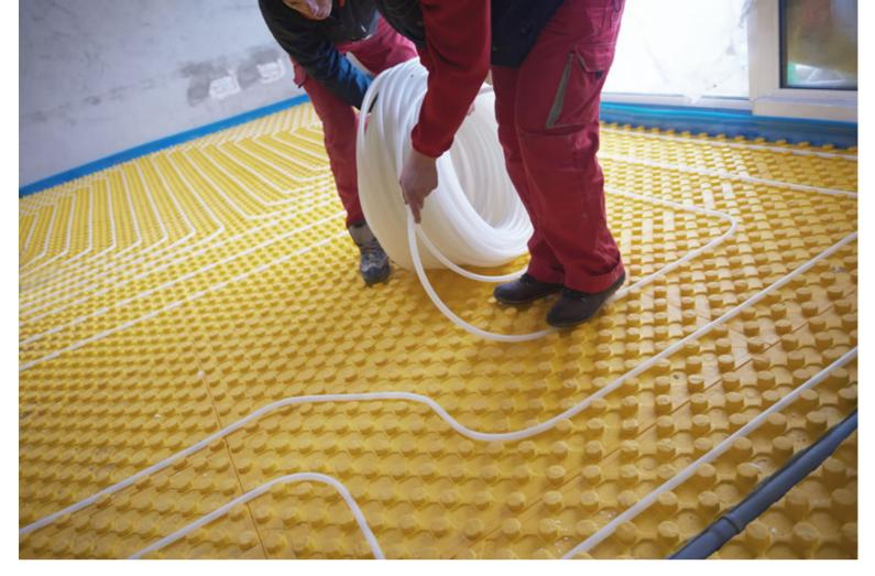
PEX pipes are often used for a speedier installation of heating in new buildings, including underfloor systems.
