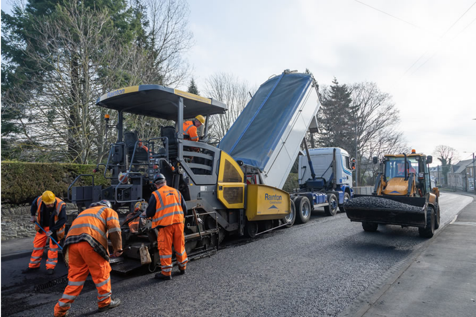
Paving the MR-based asphalt mixture. Photo: macrebur.com.
