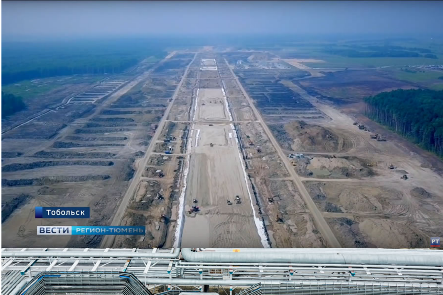
Tobolsk airport, where SIBUR is building a new runway.
