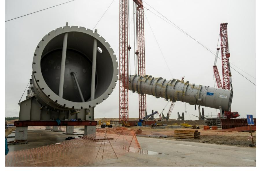
A total of 41 large-sized pieces of steam cracking equipment are scheduled for installation at the Amur GCC in 2021, 13 of which are columns
