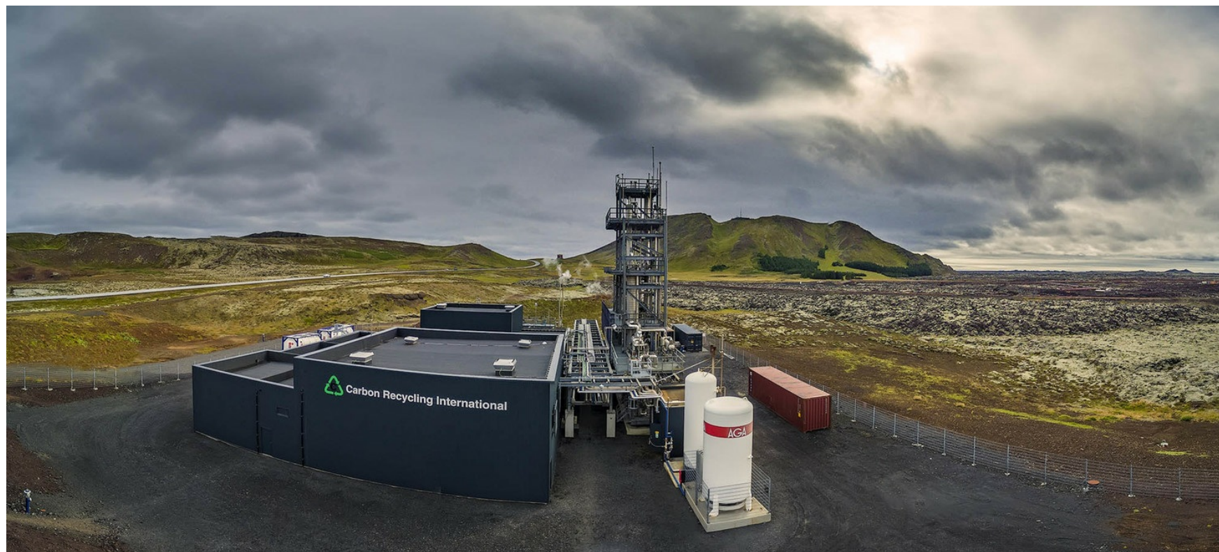
Carbon Recycling International (Iceland) developed a method to simplify the transformation of CO 2 into methanol. Photo: carbonrecycling.is
