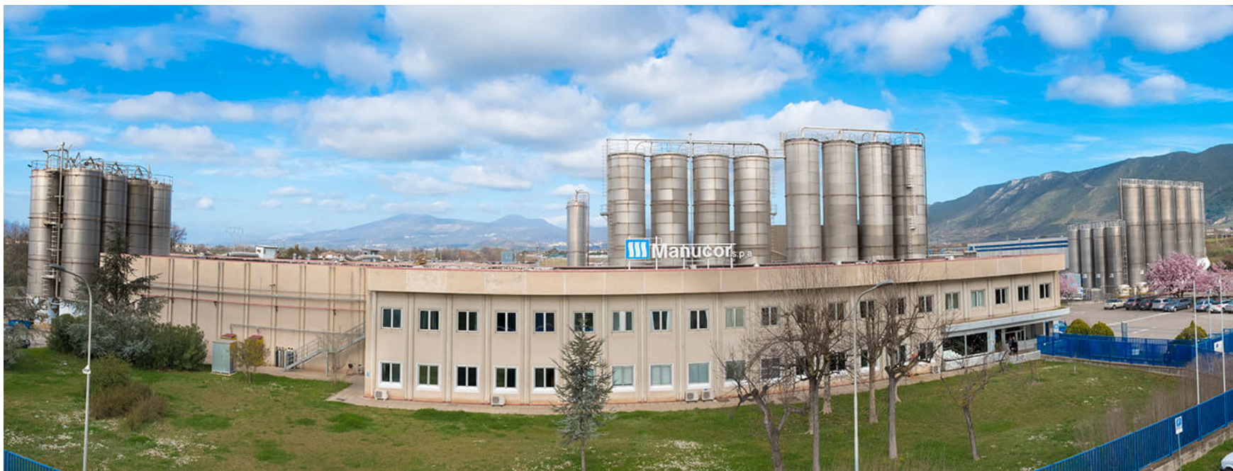
Manucor plant in Italy with a capacity of 100 ktpa of BOPP film. Photo: manucor.com.
